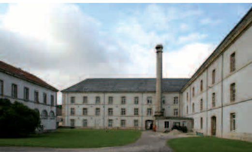
Manutention (Photo P. Thomas)
